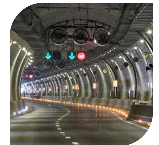
July 3rd Tunnel Port Said
